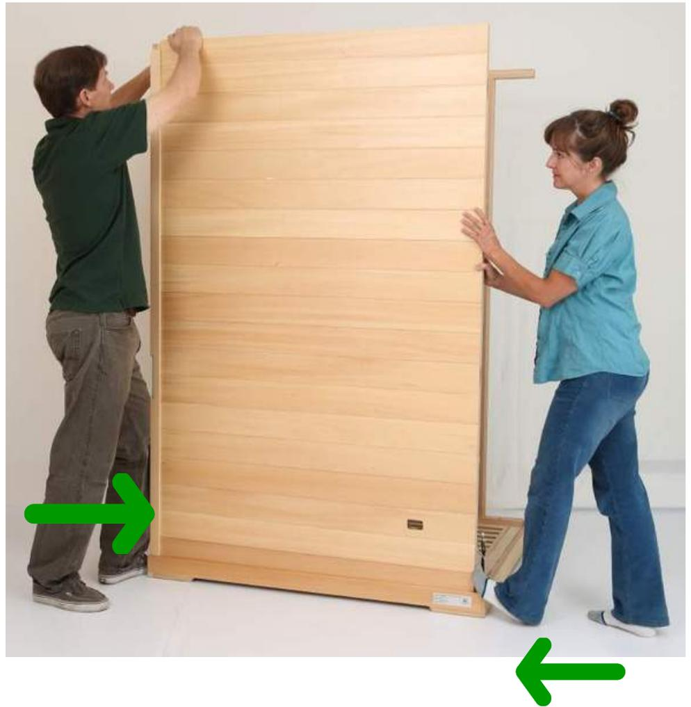
It is helpful if a second person applies pressure against the opposite edge of the back wall. This will help ensure that the two walls remain in contact and the fasteners will connect.
