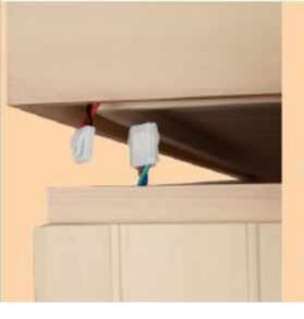
Connect the 12 Volt power supply wire at the back left corner of the sauna.
