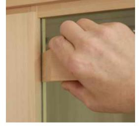
Small wooden block (included) can be used to fully press the glazing strip into channel
