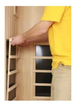
Reinstall the side wall heater guards
