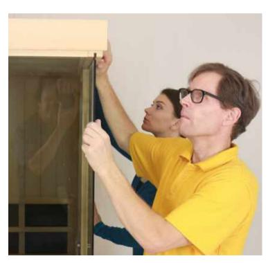
Carefully tilt the front edge of the Roof upward, about 1/2", just enough to tilt the Front Wall Glass in to position
