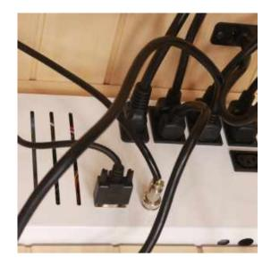
Feed the main power supply cord in through the hole in Back Wall and insert in power supply box. Do NOT plug power cord into your wall outlet until all electrical connections are finished inside of the sauna.
