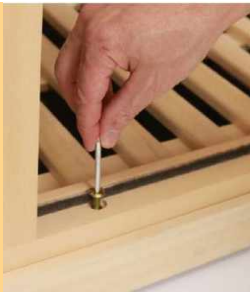
Install the 4 furniture bolts through top and bottom of door frame using the included allen key
