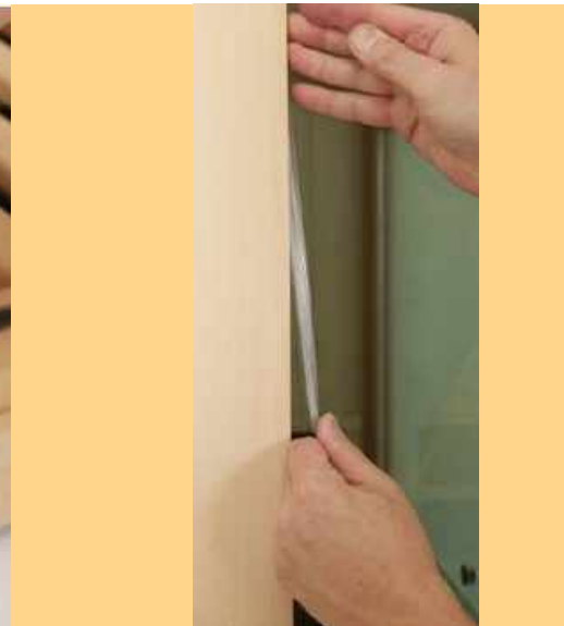
Install the remaining 2 Glazing Strips into the Right and Left Side Walls alongside the glass panels
