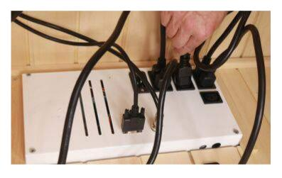
Plug in all heater leads to the receptacles in the Power Supply Box.
