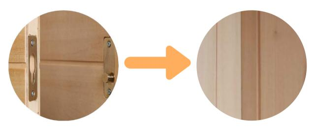
There are two sets of fasteners to join the saunas' corners together. After lowering the front wall, check to ensure that both sets of fasteners have connected by looking at the corner inside of the sauna. It is possible to connect one set of fasteners and miss the other. If there is an obvious gap in the corner between the two walls the fasteners have not connected and the raising and lowering procedure will need to be repeated.
